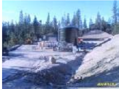
New Treatment Plant.
