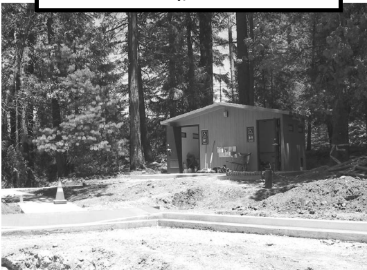
New restrooms and sidewalk
