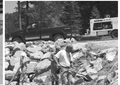
Concrete work underway
